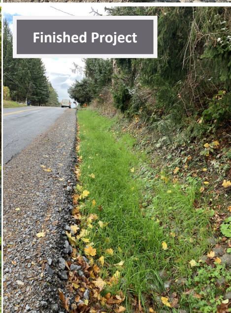
After installation is complete, the Flexamat material is then hydroseeded for further stability
